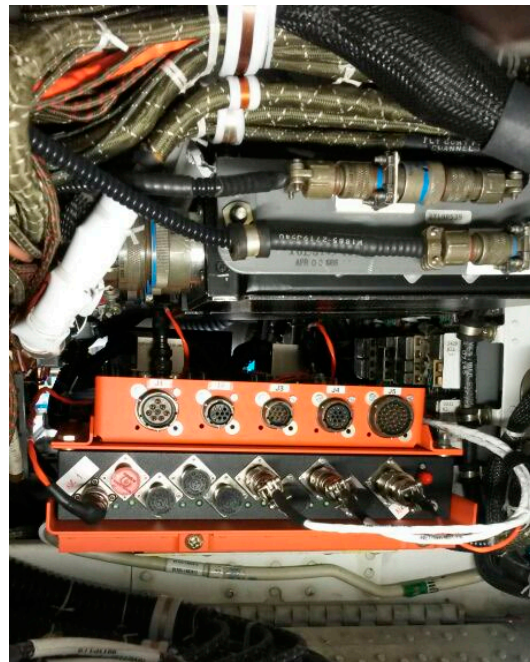
Figure 16: Installation of the master switch unit.
