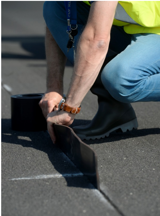
Figure 5: Flexible rubber strip in a runway groove.
