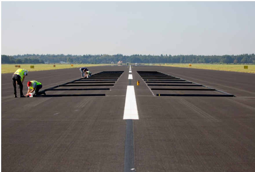
Figure 7: Water pond at Twente airport.
