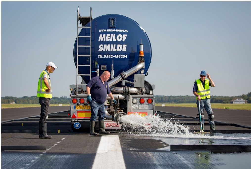
Figure 8: Filling of the water pond.
