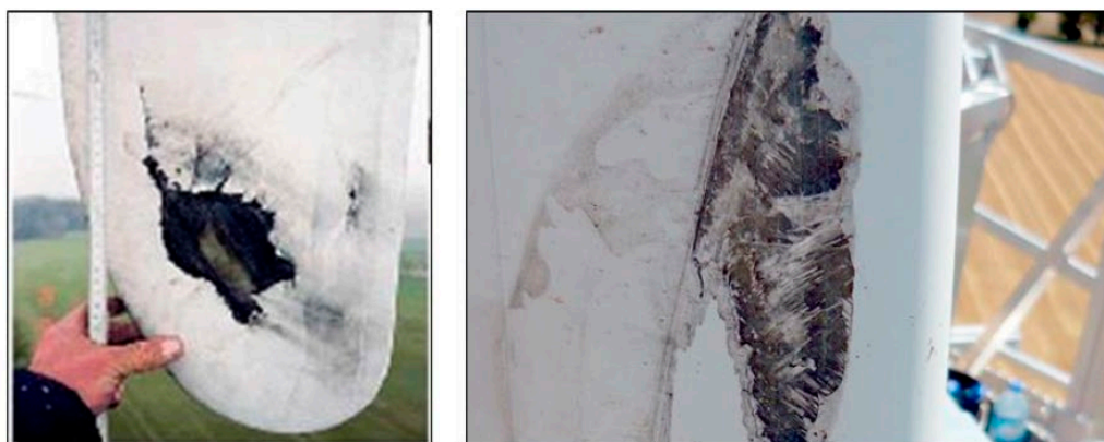
Lightning Strike Damage
