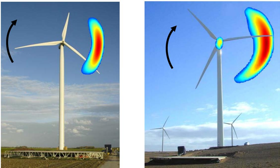
Figure 2: GE 2.3 MW turbine (left) and GAMESA 850 kW turbine (right) with typical noise source distribution in the rotor plane.
