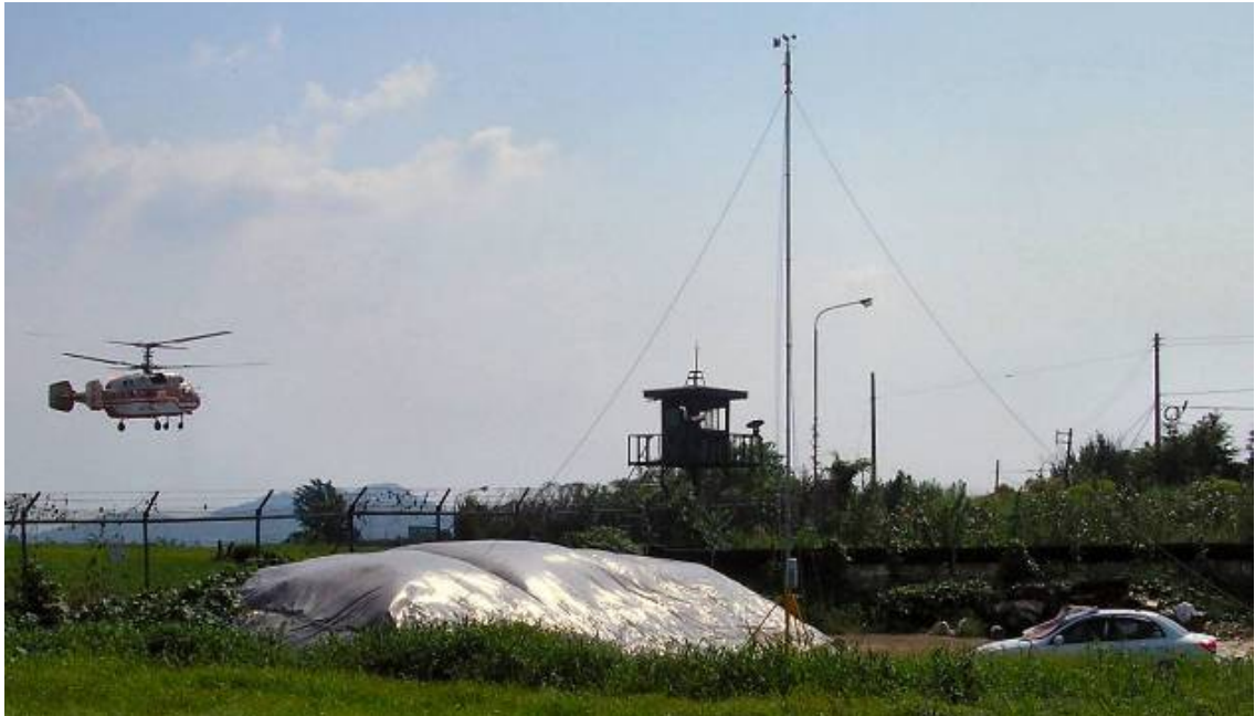
Figure 10: Installation site of meteo mast at Jeonju air force base
