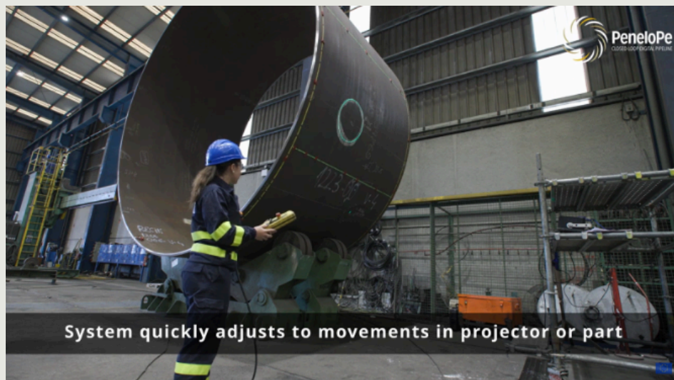
Figure 8. Adaptive projection for insite tracing of auxiliary elements in large components.
