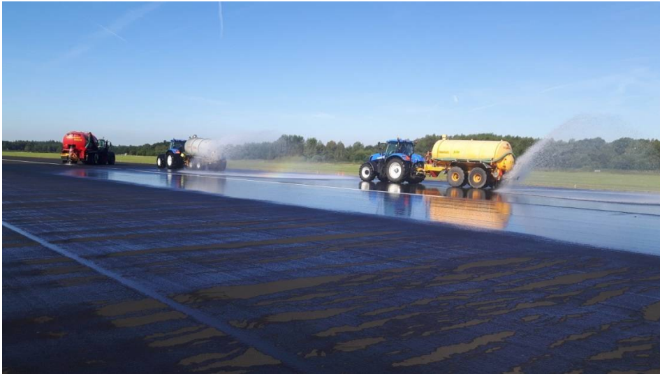
Figure 1: Tests to determine amount of water required to wet the runway.
