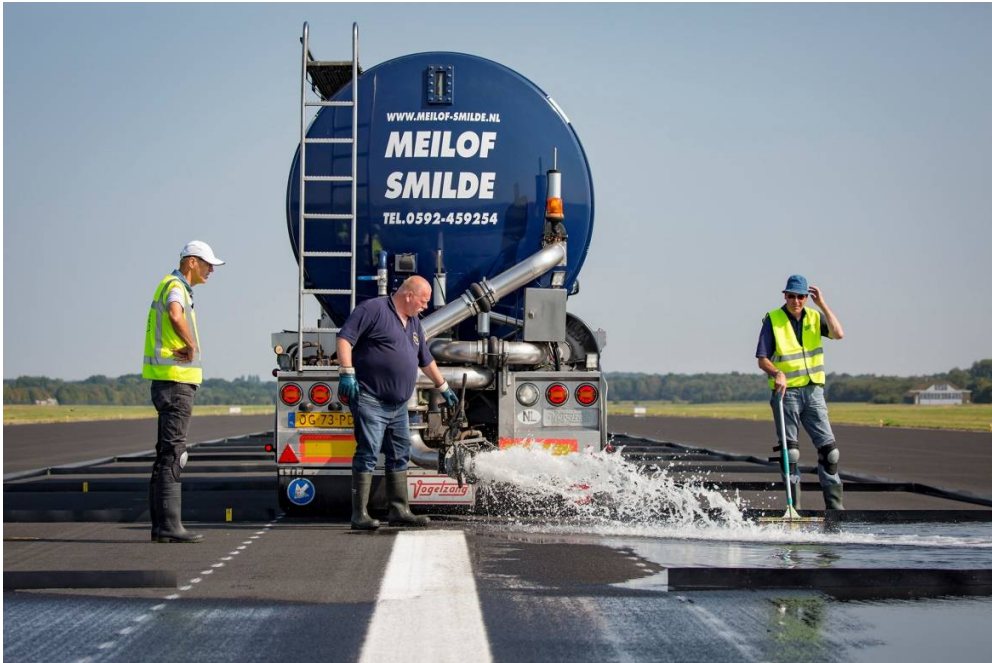
Figure 13: Filling of the water pond.
