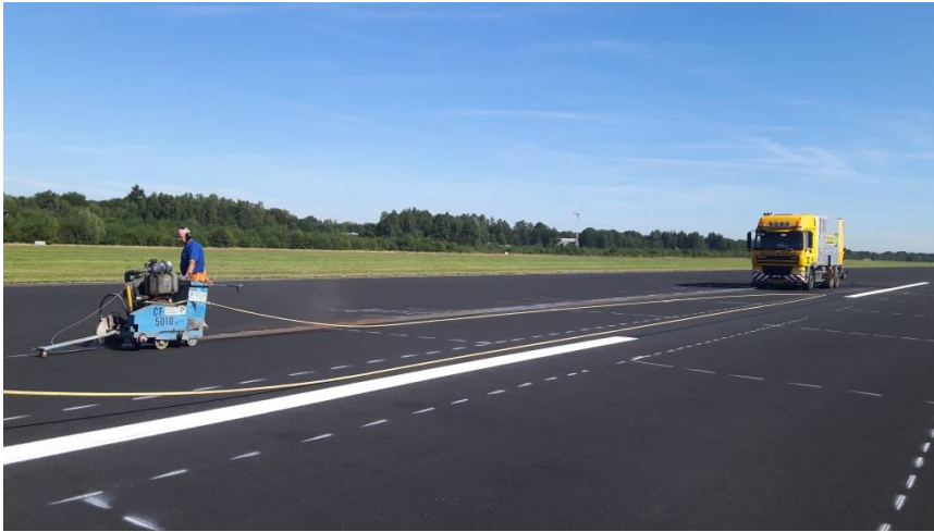
Figure 11: Construction of grooves into the runway for the water pond.
