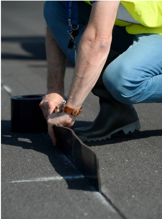
Figure 8: Flexible rubber strip in a runway groove.
