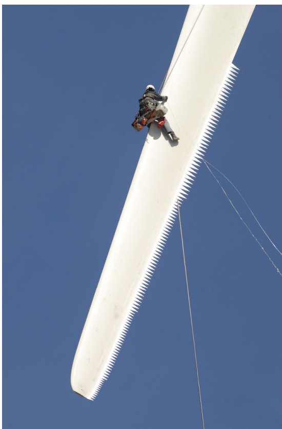
Figure 42 Climber removing trips from serrated blade
